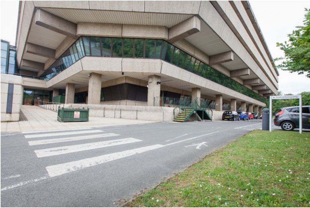
Figure 3. View of accessible parking bays and rear entrance ramp
