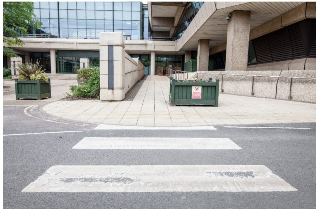
Figure 4. View of rear entrance ramp from accessible parking bays
