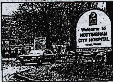
TESTS AND CHECKS: Nottingham City Hospital
